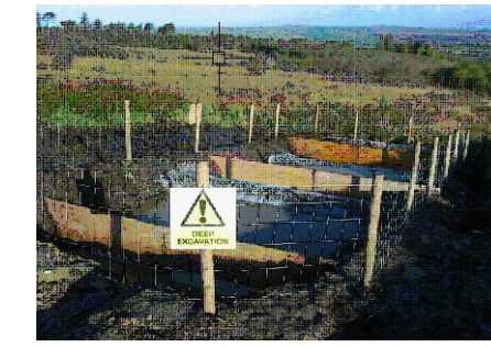
COMPLETED SETTLEMENT POND SYSTEM N.T.SCALE
